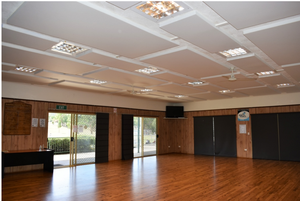
White Calando Panel applied to the Hodgson Vale Community Sports Club Ceiling.
