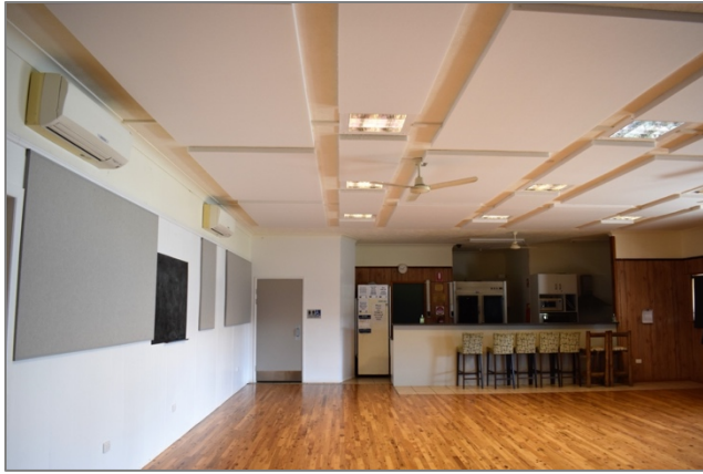
Calando One Panels for the wall helped improve the acoustics.
